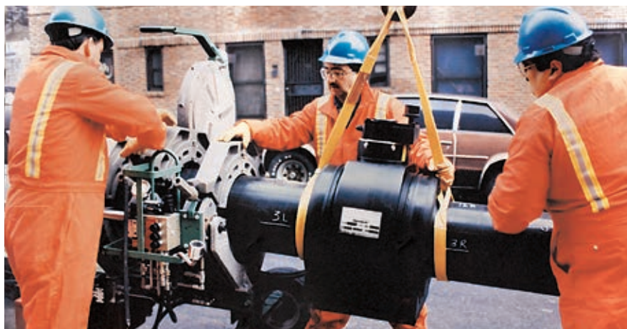
12" Poly-Gas® valve fusion operation
