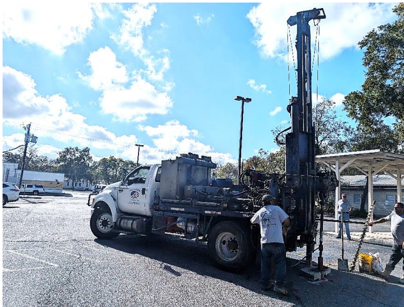
Photo 2 – View looking at drilling of boring P-5
