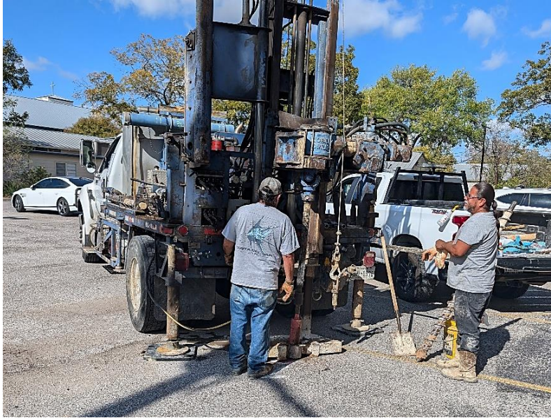
Photo 1 – View looking at drilling of boring P-1
