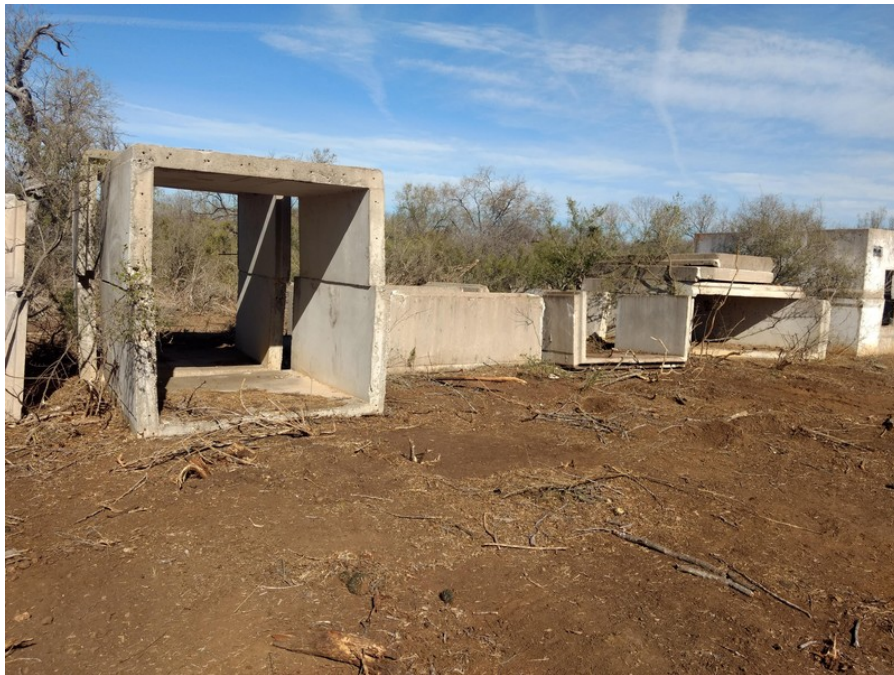
Photo 8: View of large concrete pieces on the east central portion of the subject site.
