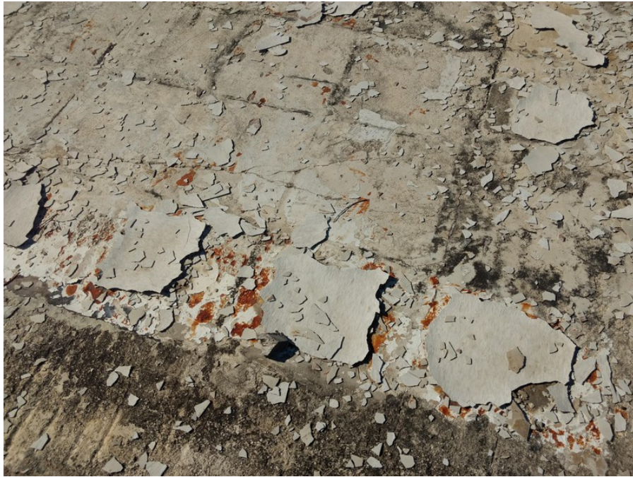
Photo 27: View of remnants of tile on the previously pictured concrete slab.
