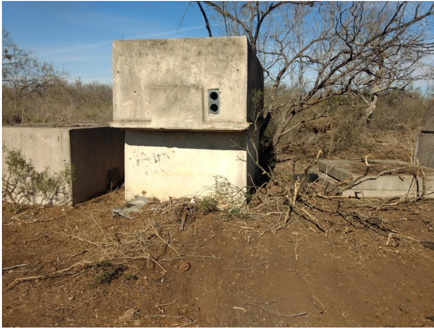
Photo 9: Another view of the large concrete pieces on the east portion of the subject site.
