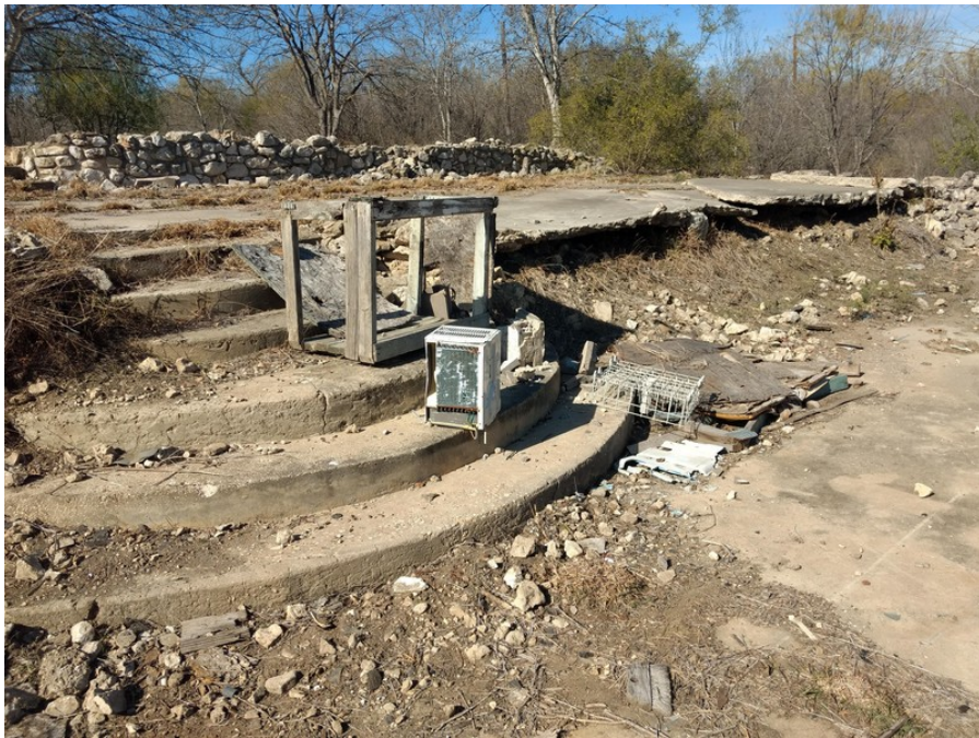
Photo 26: View of a vacant concrete slab on the northeast portion of the subject site.
