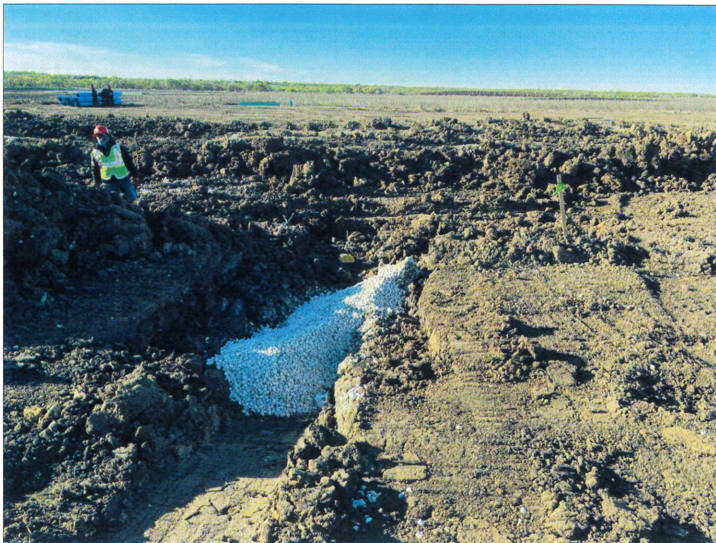
Lot 43 tested 6" sewer lateral
