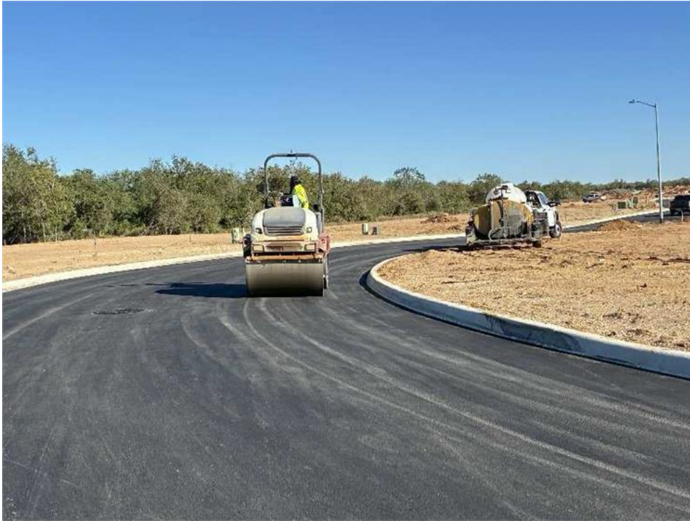
Compaction in progress
