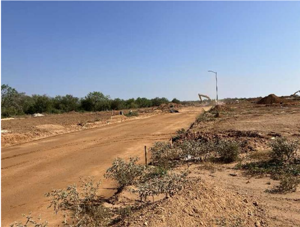
Quartz cove lime treated subgrade near station 11+00
