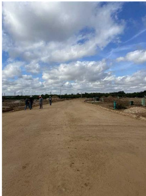
Compacted base preparation for testing on Mudstone Pl.
