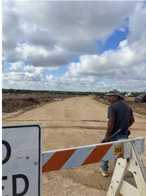
Compacted base at the beginning of the Mudstone Pl. section, prior to testing.
