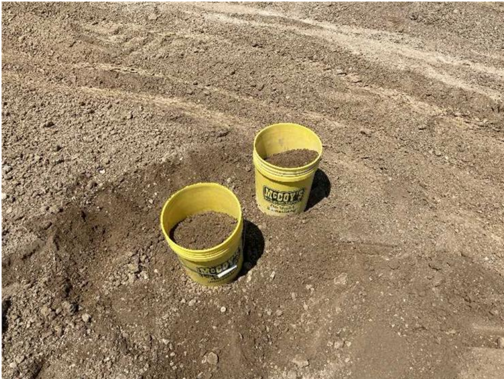
Lime treated subgrade at Bassalts Garden near station 1+00
