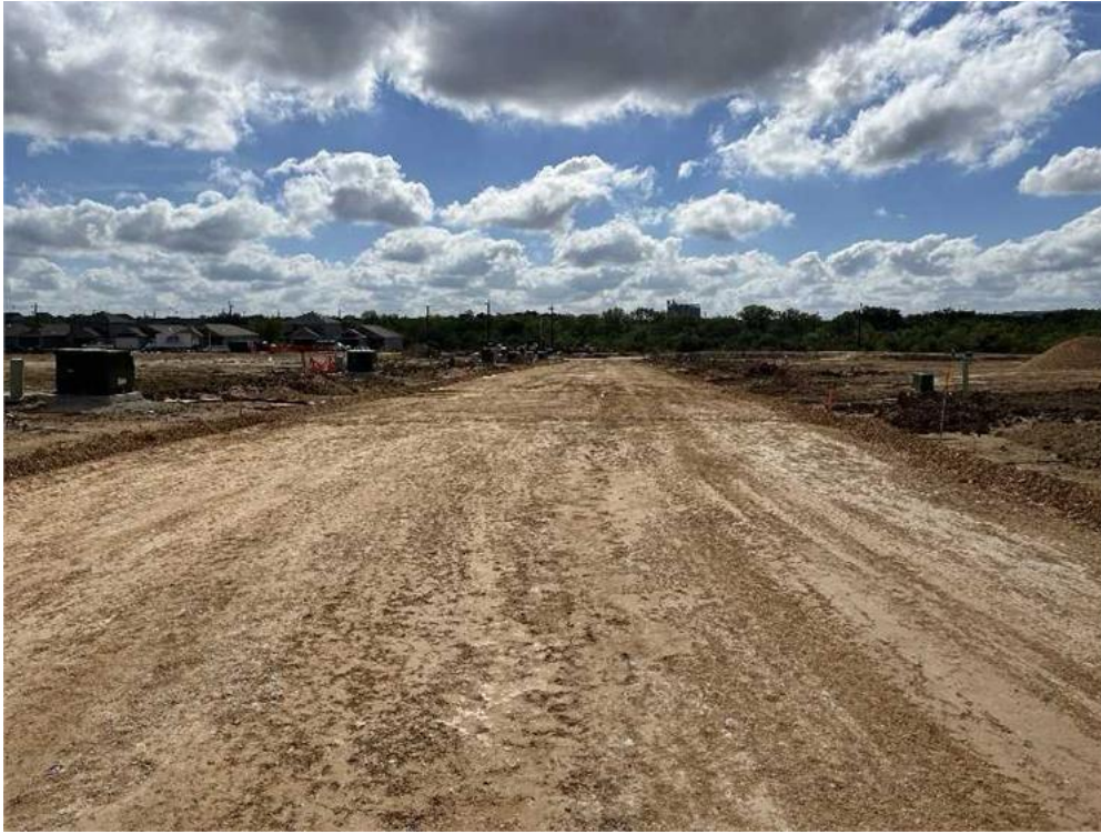
View of flexible base processing in progress, Chalk Cave.
