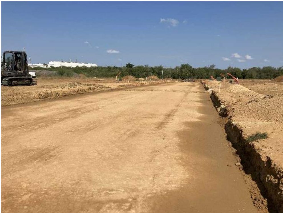
Dacite Place like treated subgrade near station 2+00
