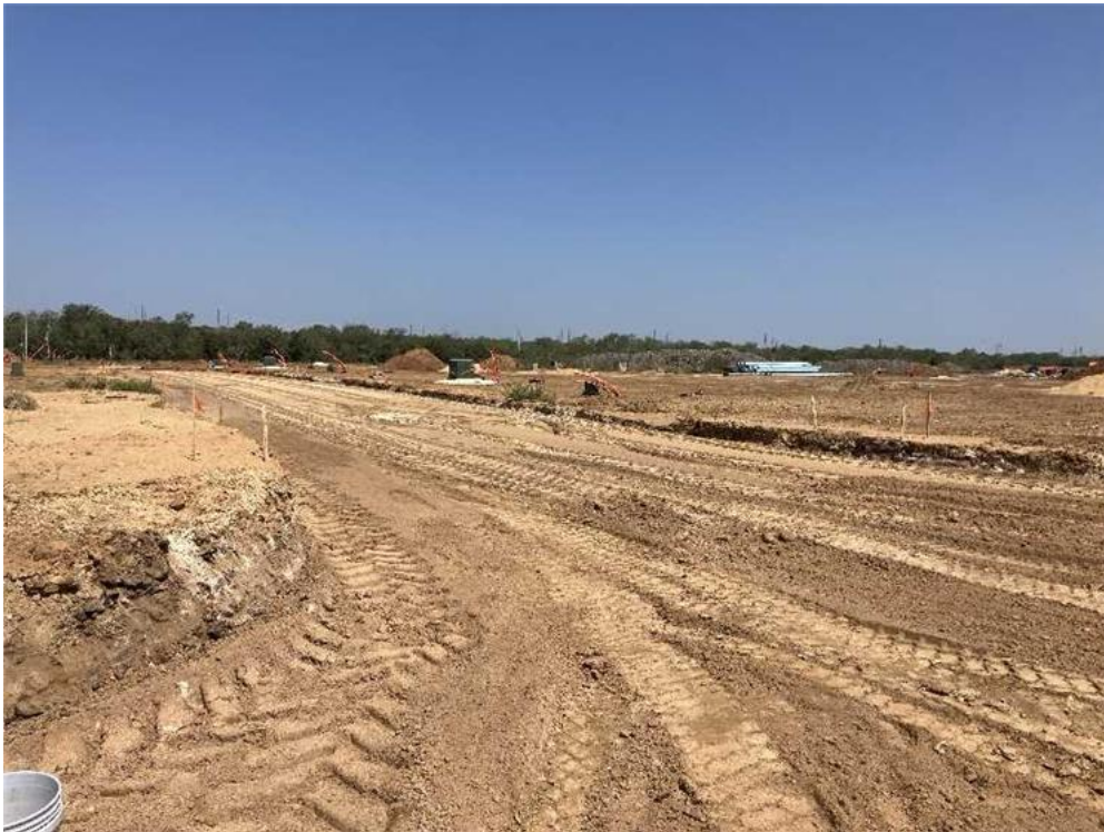
Dacite Place appears to be mixed with lime prior to gradations and sampling
