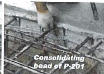
Applying bead of P-201
