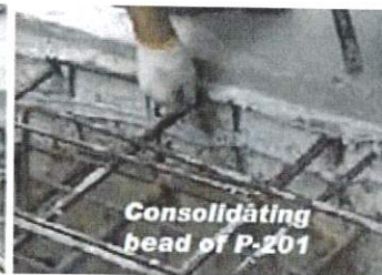
Applying bead of P-201
